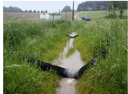
Runoff from a field planted with corn is directed into a grassed waterway where it passes through and over a series of compost-filled filter socks that help reduce levels of nutrients and herbicides. (D1326-1)
