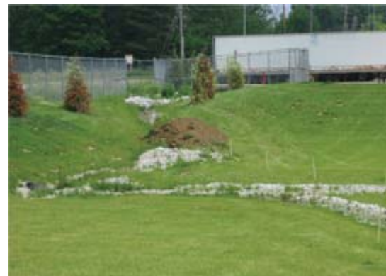
Hormel Foods' original detention basin met only basic flood control requirements.
