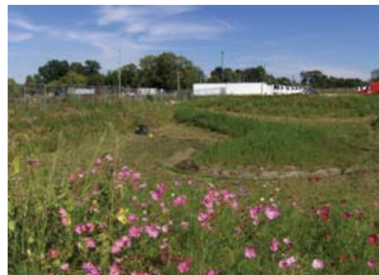
Fescue eradication and sideslope stabilization are key benefits of the finished project.
