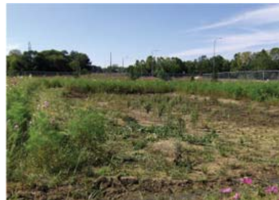
Redesigning the basin included the establishment of a 4,500-square-foot rain garden.
