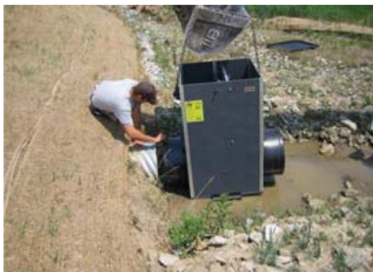
A water control device on an existing detention basin outlet
