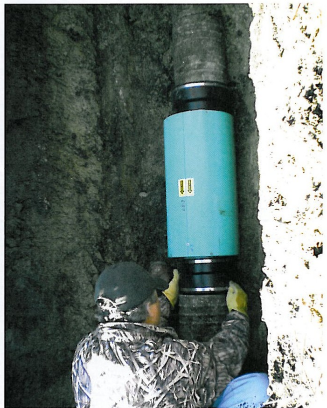
Installing remotely controlled in-ground control structures could make drainage water management feasible on millions more acres of farmland.
