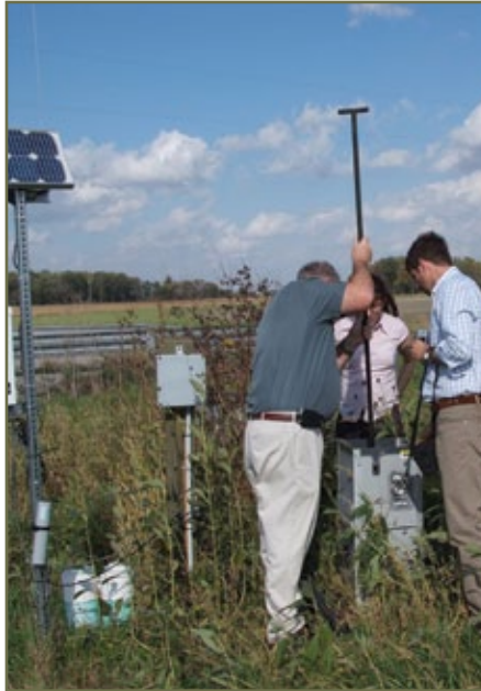
Leonard Binstock of the Agricultural Drainage Management Coalition adjusts stop-logs in one of Doug Mills' control structures.
